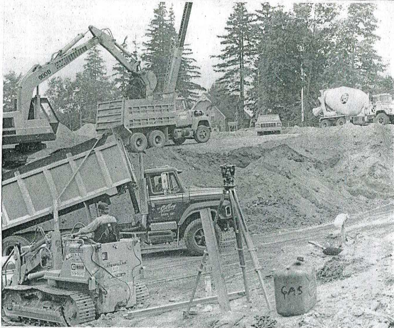
LOTS OF ACTIVITY — There were many machines at work at the Ayr apartment complex last week. Workmen had to dig out a pocket of black muck and replace it with gravel. Another crew was forming the footings and had two concrete trucks in place ready to pour when they discovered that reinforcing rod had not been delivered. On Monday workers were putting the rod in place and pouring concrete footings.
